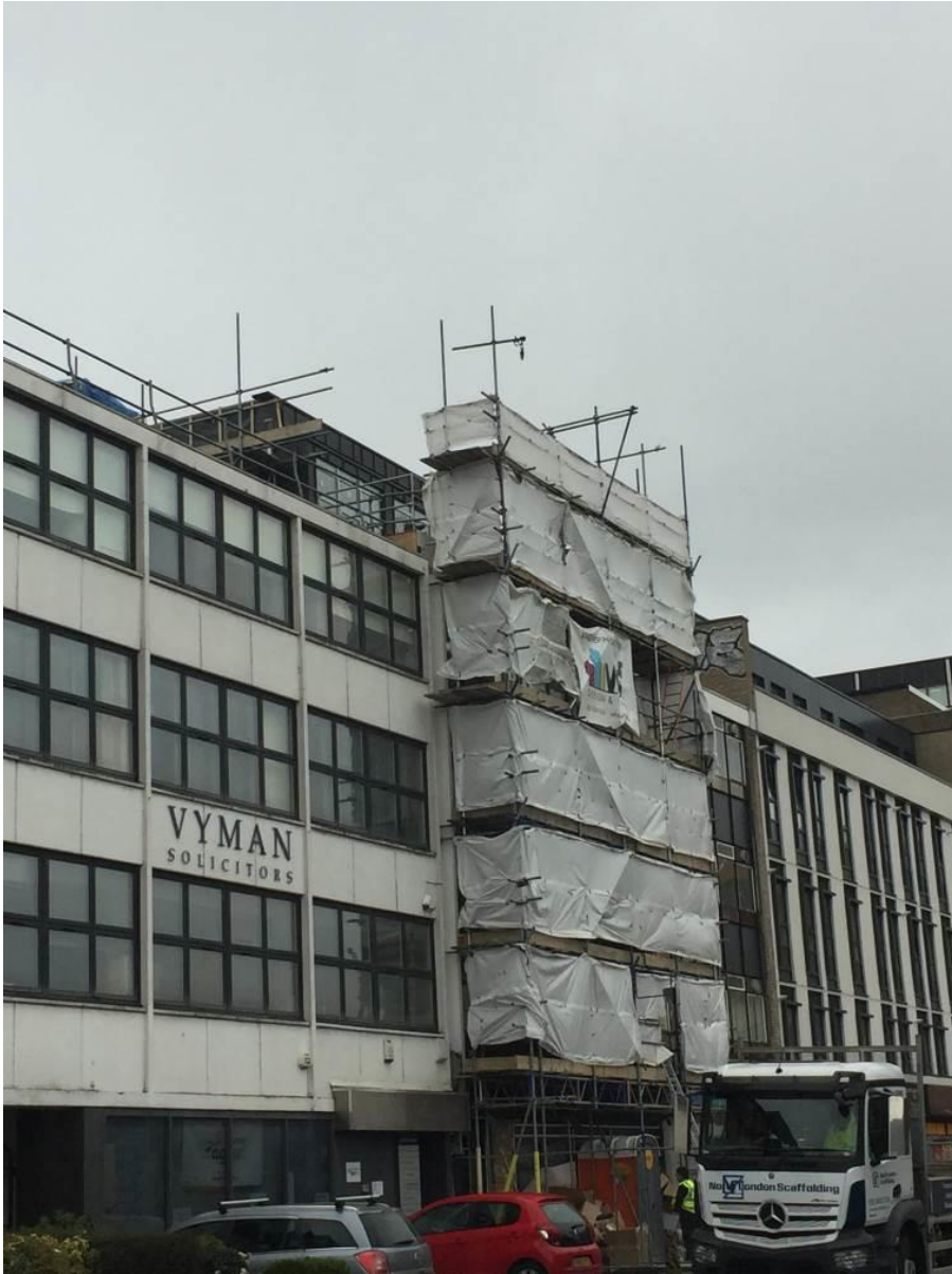
Detail showing recently built 4 th floor
