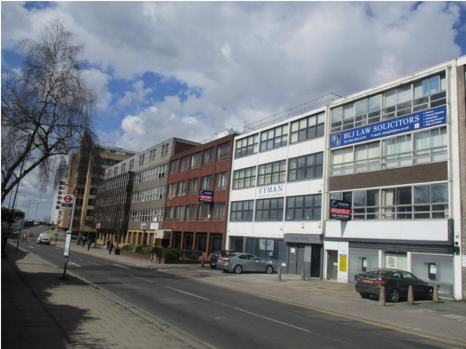
Pre-existing building – front elevation
